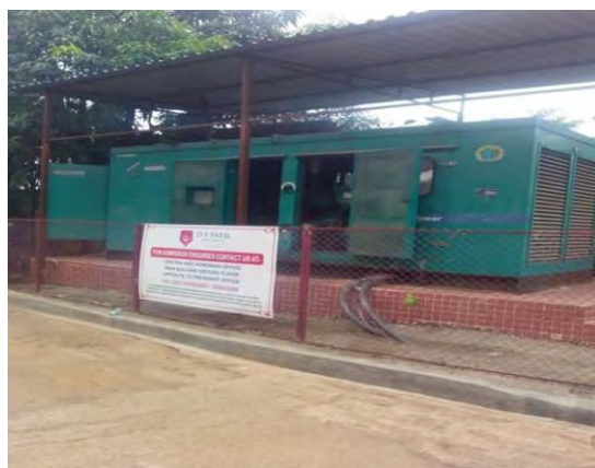
Fig. 4.37: Generator, power supply unit.
