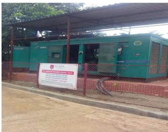
Fig. 4.37: Generator, power supply unit.
