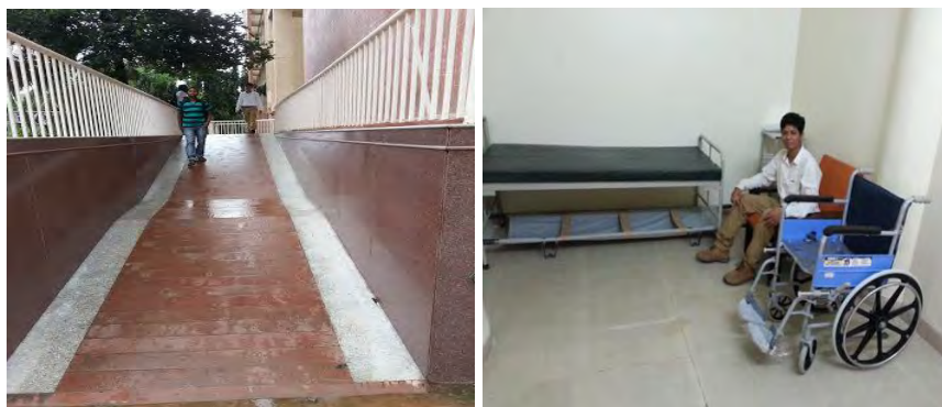
Fig. 4.22: Ramp, wheel chair and stretcher facility.
